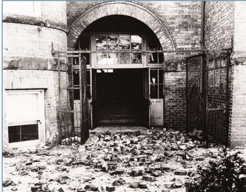
Figure 4-22 Another dangerous entry collapse, Seattle, WA, 1949
