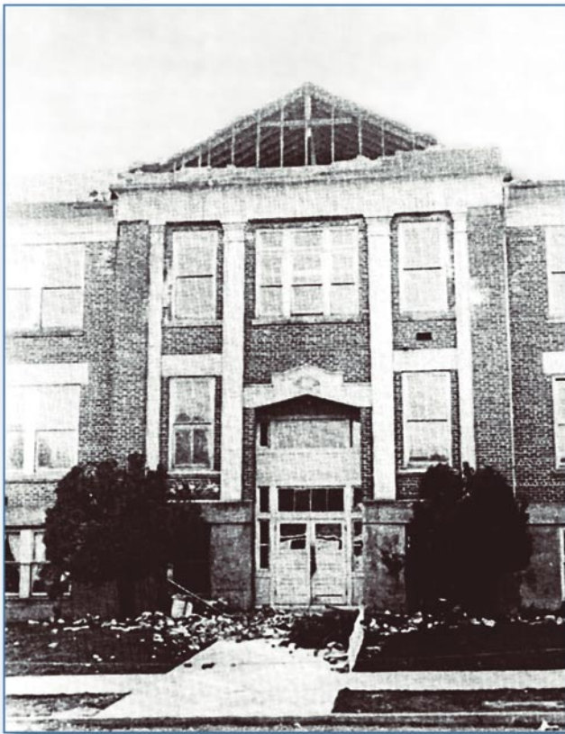
Figure 4-21 The student body president was killed here by falling brickwork, Seattle, WA, 1949.
