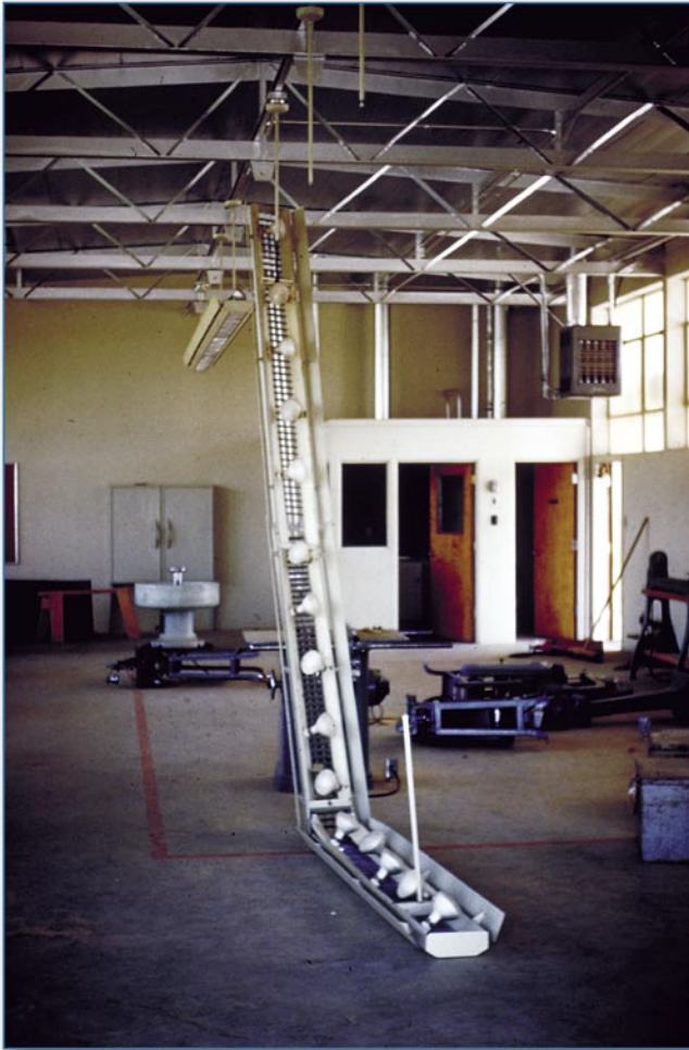
Figure 4-18 Overturned shop equipment and failed light fixtures, Kern County, CA, 1952
