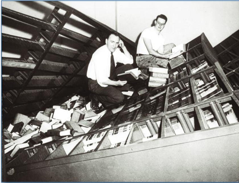
Figure 4-24 Damage to library shelving, Seattle, WA, 1949
